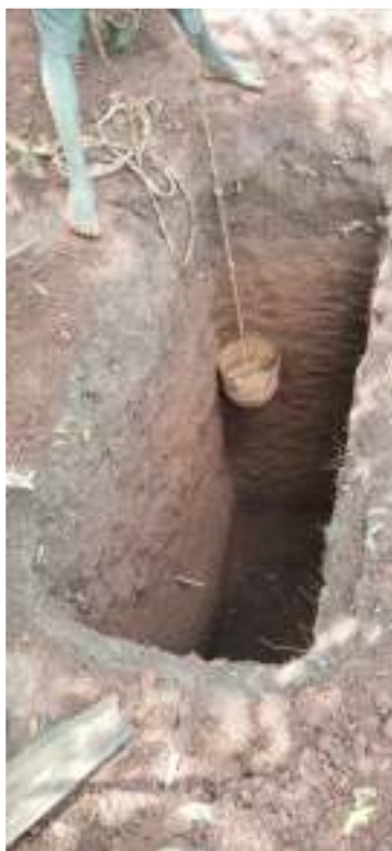
One man at the top pulling up the dirt. The other man at the bottom, digging and filling up the bucket.
