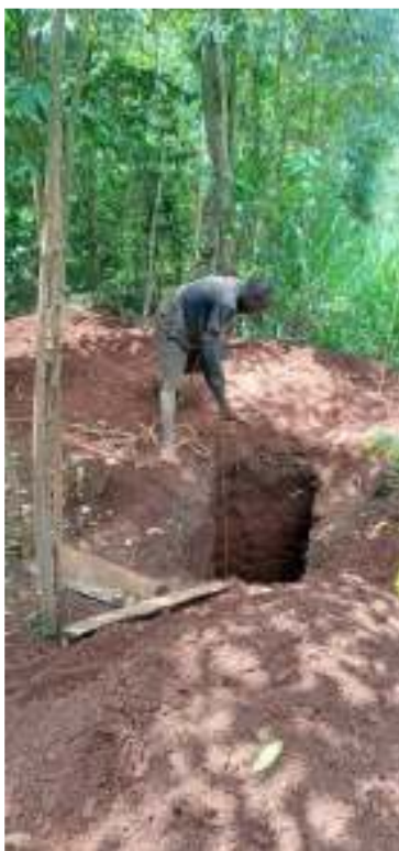
One man at the top pulling up the dirt. The other man at the bottom, digging and filling up the bucket.
